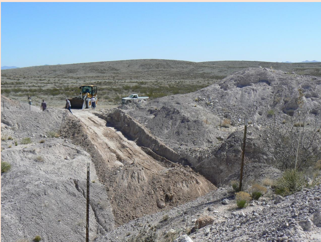
Verfüllung der Baker Egg Mine / Backfilling of the Baker Egg Mine. 2015/2016. Loren Seng photos.
